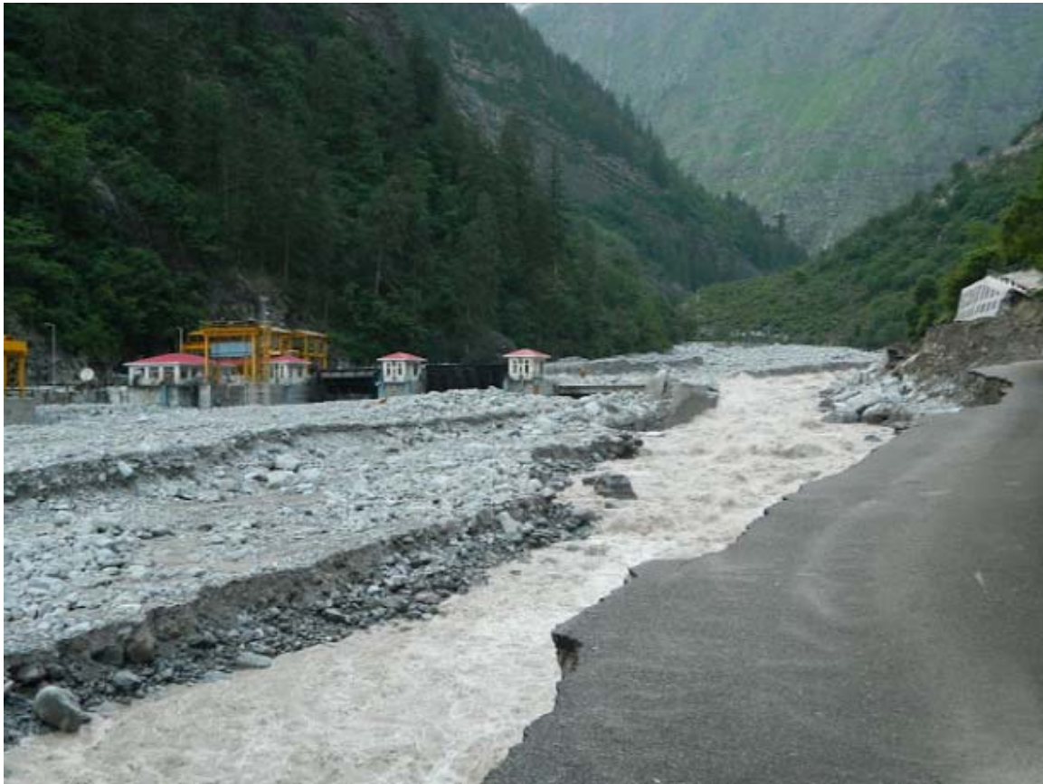
Destroyed Vishnupryag HEP (400MW), Alaknandaganga flowing on the left side, made new path for herself.
